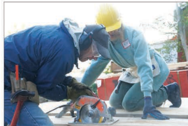
Faith Builders 2013 Blitz Build Volunteers.
